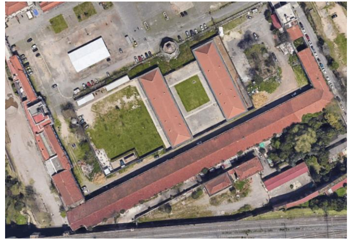
Figure 2: Satellite image of the Slaughterhouse roof
