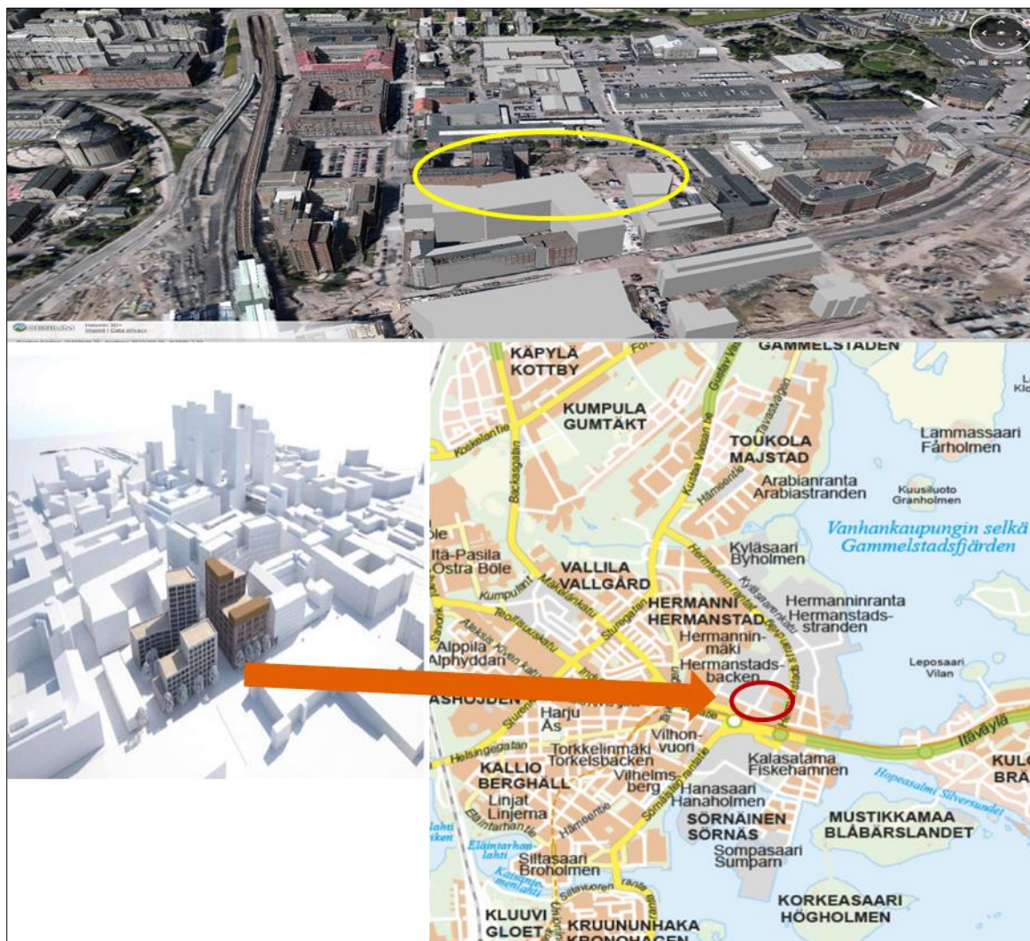
Figure 2-5: The EXCESS project demo case building location and planned area in Kalasatama, Helsinki Source: Sweco architects Oy, [2], [3].
