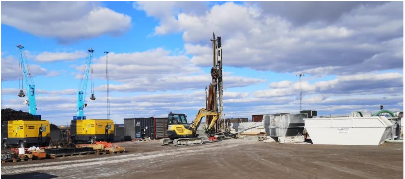
Figure 8 Drilling machinery in drill site in Malmö, (source: St1 geothermal)
