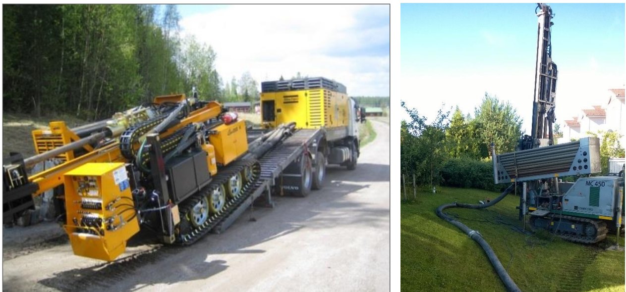
Figure 2 Typical drilling equipment arriving at the drill site
