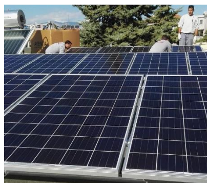
Photograph of the PV-system being installed [Source: Stefan Pallantzas]
