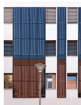
Photograph of the PV-system integrated into the façade of House 1 [Source: Andrea Kroth]
